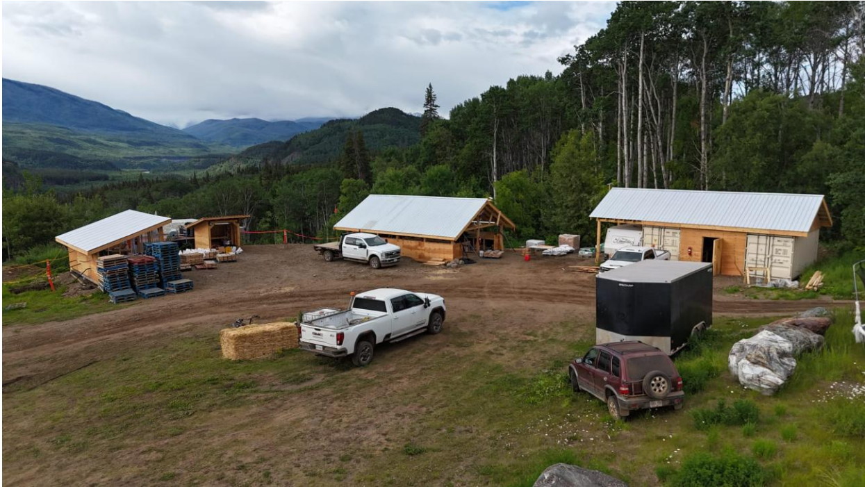
Newly built core logging facilities
